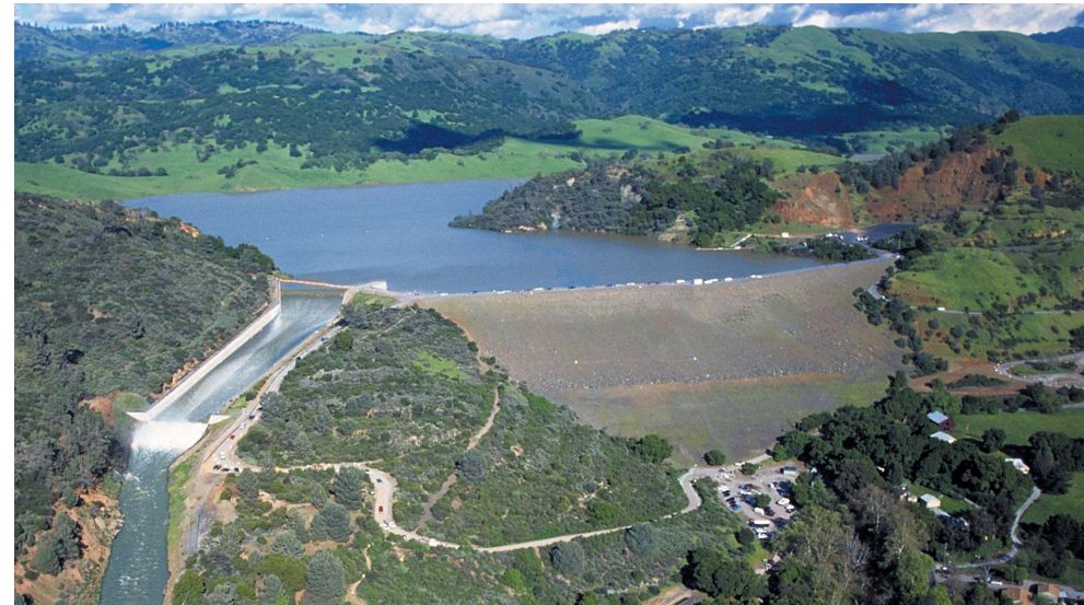
Anderson Dam, California
