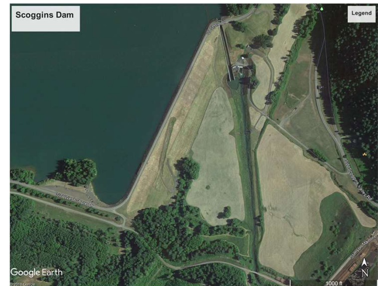
Scoggins Dam, Oregon
