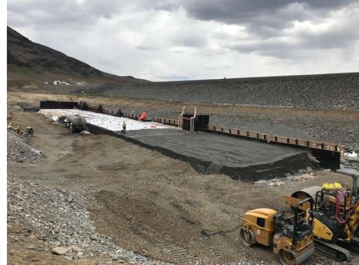
Priest Rapids Dam, Washington
