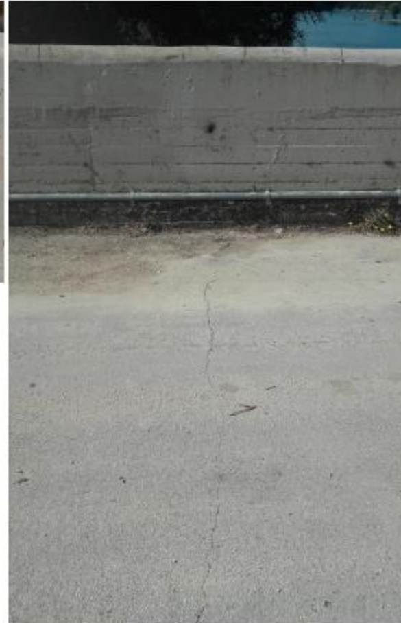
Scandarello Dam. Slight damages on the parapet and crack pattern on the crest.
