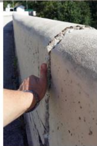
Scandarello Dam. Slight damages on the parapet and crack pattern on the crest.
