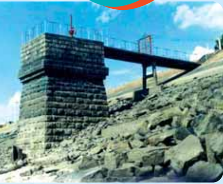
Ancient outlet tower of Minneriya dam that was built 276 -303 AD in Sri Lanka and was restored in 1901 for irrigation. It is still in use today
